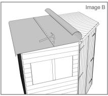
Roll the last piece over the roof and secure with clout nails. (Image C). Then pull the edge of the felt tightly over the roof and nail in place. Secure all the way around the roof.
